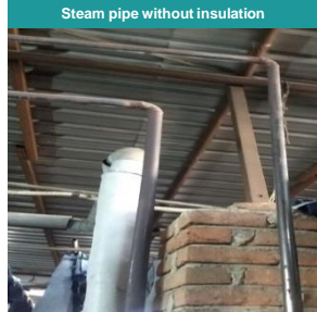
Steam pipe without insulation
